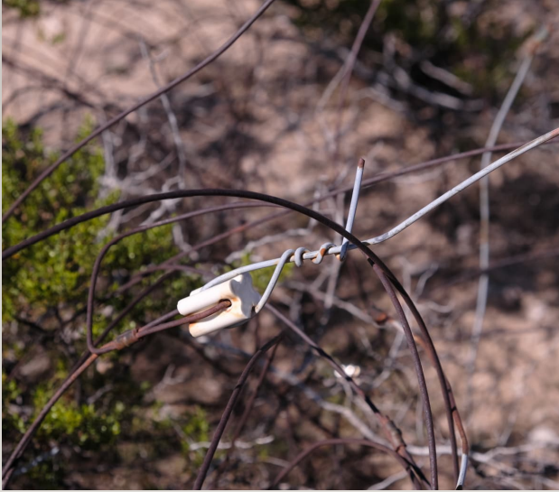
Wire and ceramic insulator, probably from the receiving array backscreen
