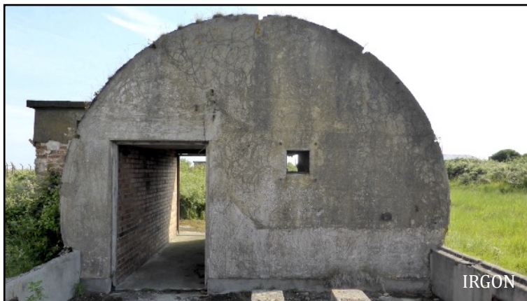
Fig 2. Internal view showing semi-circular profile was normally covered in steel sheeting. (as of 2021) Entry port for sabot/scale-model combination is visible in wall. External control room is just visible through doorway.
