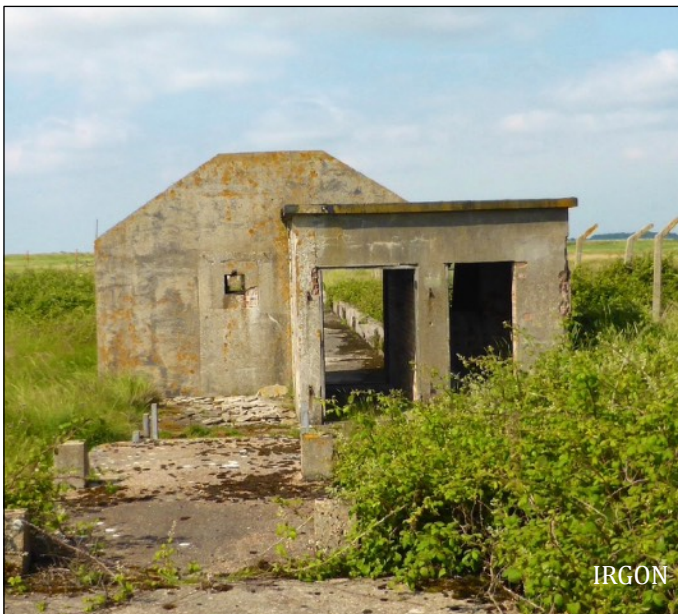
Fig 3: View of the '17-pdr' plinth and gun port location
